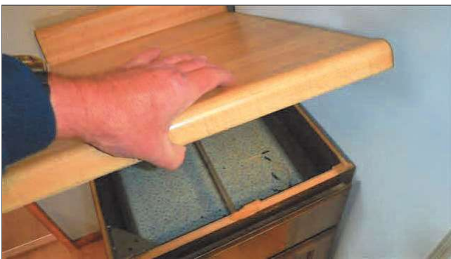
4.3 (2) The countertop could use some finishing work where it meets the wall (backsplash) and one small section of counter is very loose.
